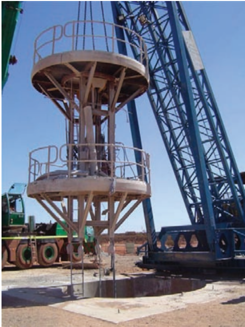
Installing the Double Deck Stage
