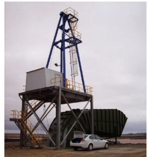
Egress System Installed over Surface Fan
