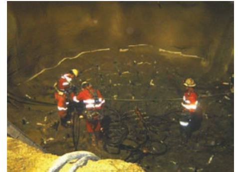
Boring the Cut in the ROM Bin
