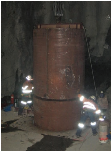
Ore Bin Wear Liner
