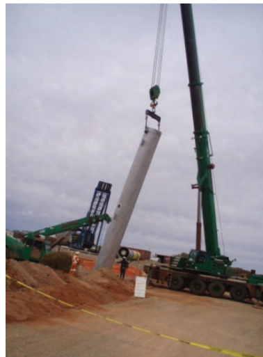
207m Long Egress Ladderway
