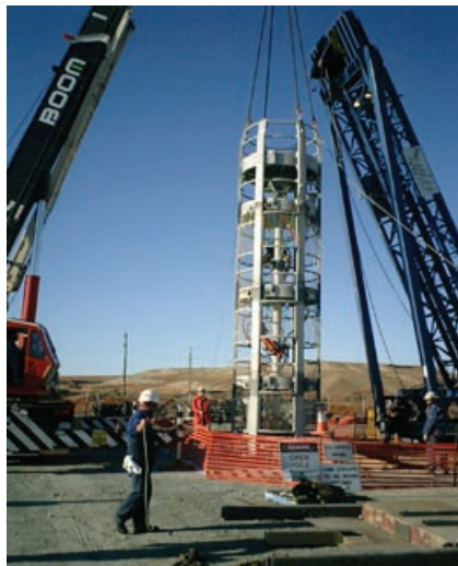
Installing the Horidiam Stage
