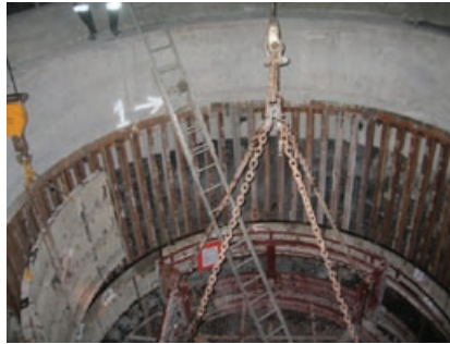
Fine Ore Bin Rail Liner Installation
