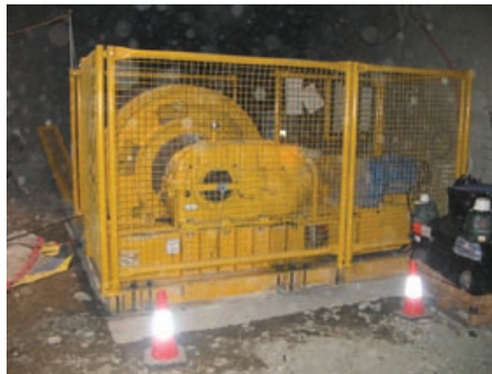
Underground Hoist Installation
