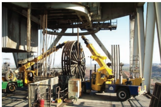
Installing the sheaves in the Headframe
