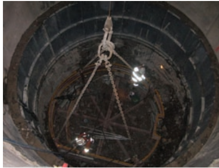
Installing Formwork in the Vertical Dam
