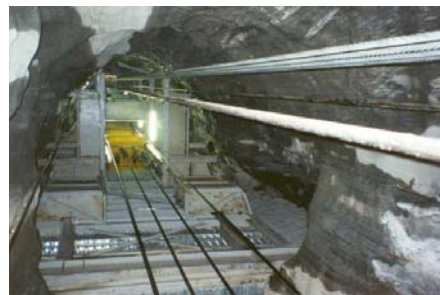
Renison Internal Haulage Shaft
