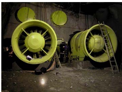
Underground Fan Installations
