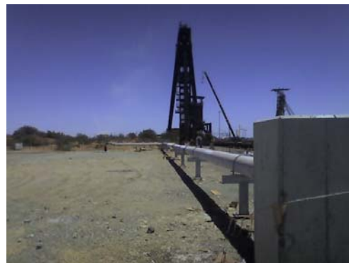
2.5 Kilometres of Compressed Air line installation
