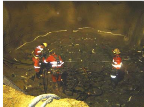
Boring the Cut in the ROM Bin
