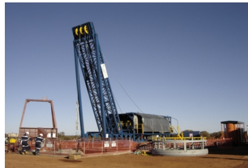
Headframe Installation
