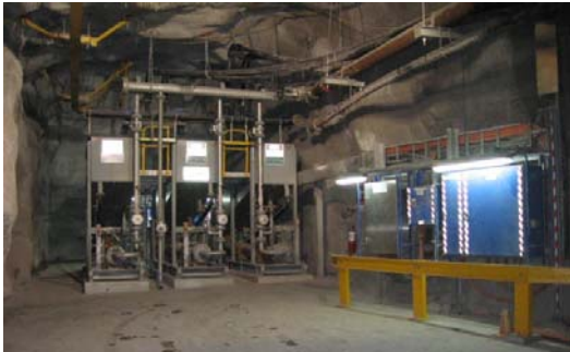
Underground Pump Station
