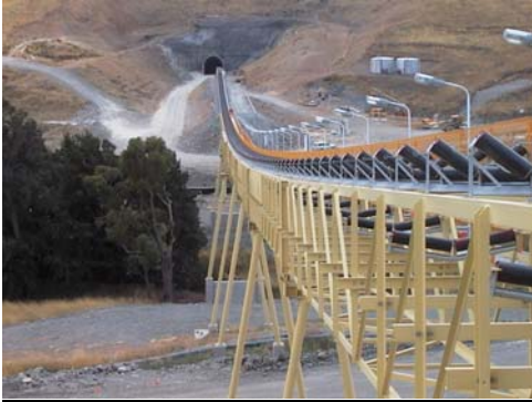
Ridgeway Mine Conveyor Installation
