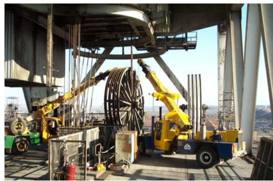
Installing the sheaves in the Headframe
