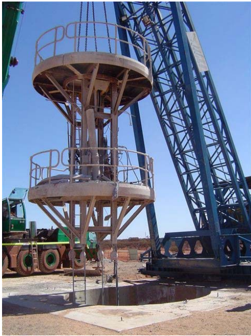
Installing the Double Deck Stage
