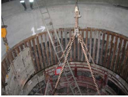
Fine Ore Bin Rail Liner Installation
