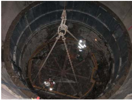
Installing Formwork in the Vertical Dam
