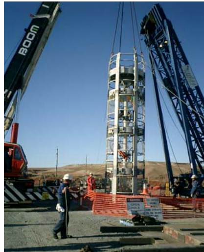
Installing the Horidiam Stage
