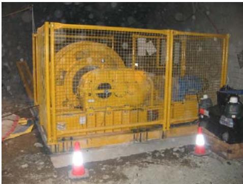
Underground Hoist Installation
