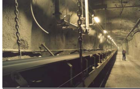
North Parks Underground Conveyor Installation
